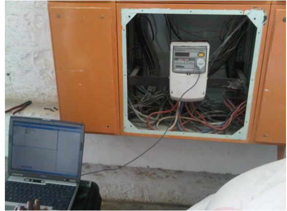
Figure 4.18: Down loading of data -Submeter Powder Section
